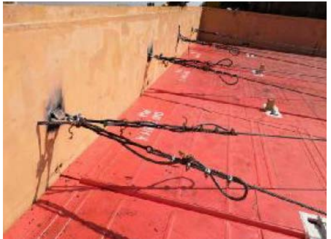
Cable lashing connected by Turn Buckle
