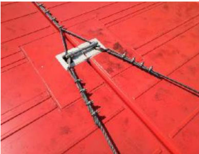
Bridge fitting securing position
